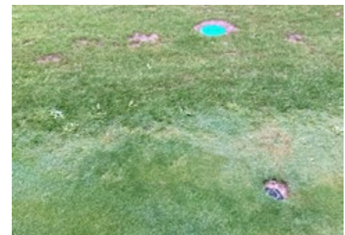
Re-installing the lawn tiles to cover the sensors. 14 days later - "invisible"
