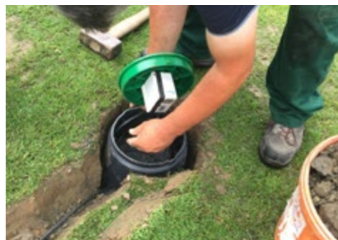
Preparation of the irrigation box for the data logger
